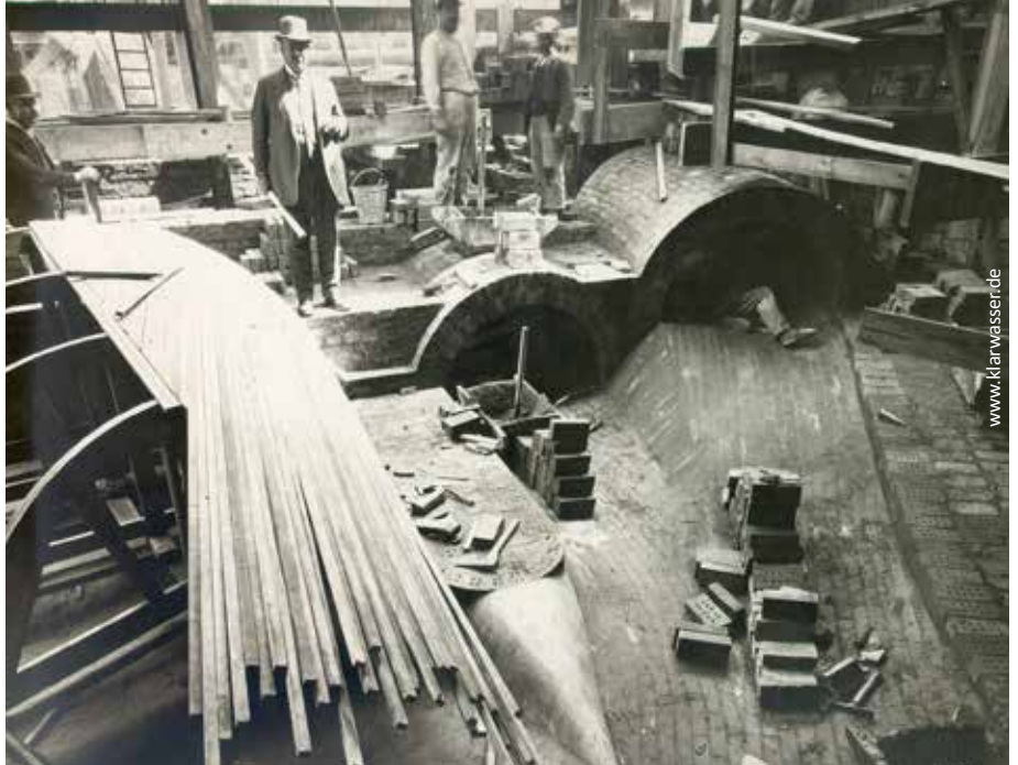
Construction of the sewage radial system in Berlin. Since 1878 the waste water of the City was sent to sewage fields outside Berlin and no longer in the Spree.
